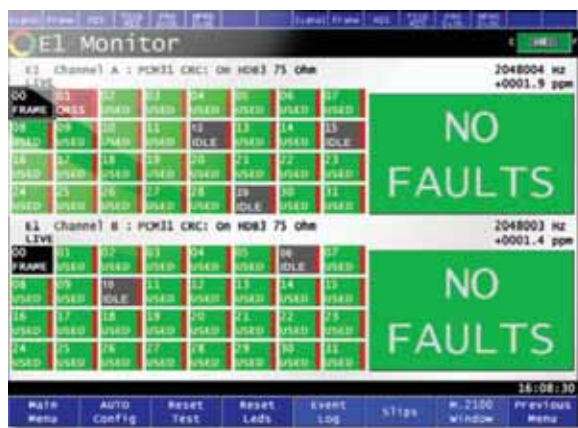
Monitoring a Live E1 Circuit
